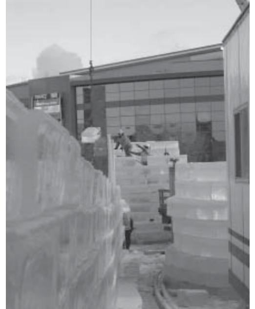
Builders with flame throwers construct one of the Ice Palace walls - above . Below - Construction site of the 2004 Ice Palace
